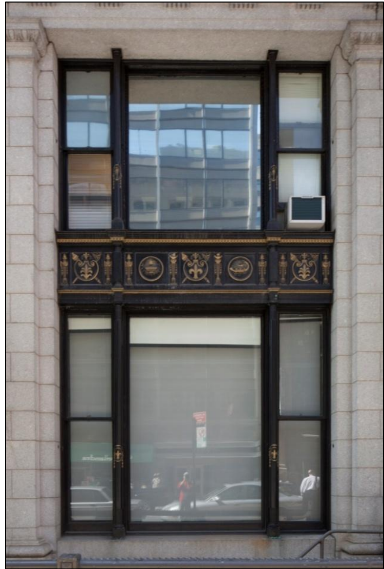
Brooklyn Union Gas Company Building Bronze window panels of main story Photo: Christopher D. Brazee (2011)
